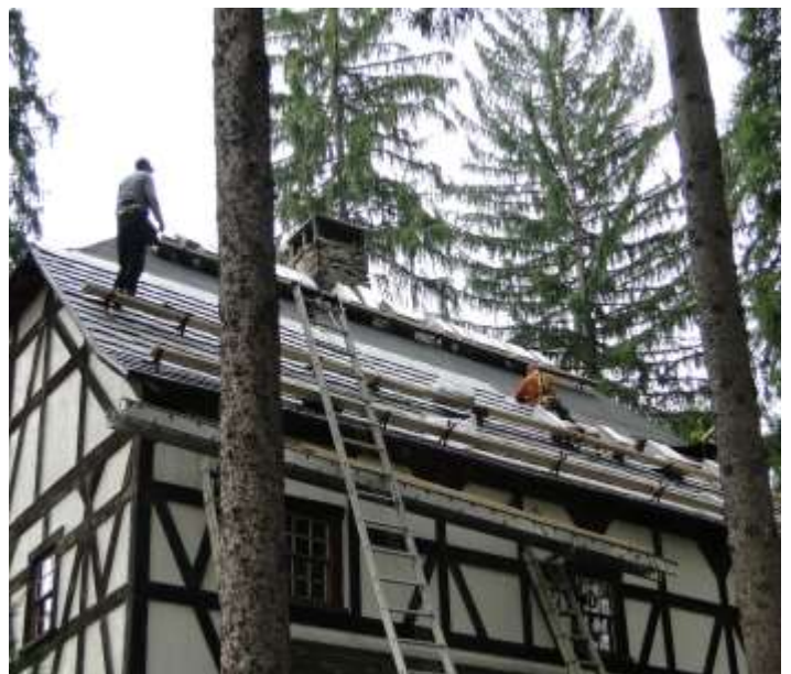
Knotts Construction, Ridgeley WV, replacing the shingles.
